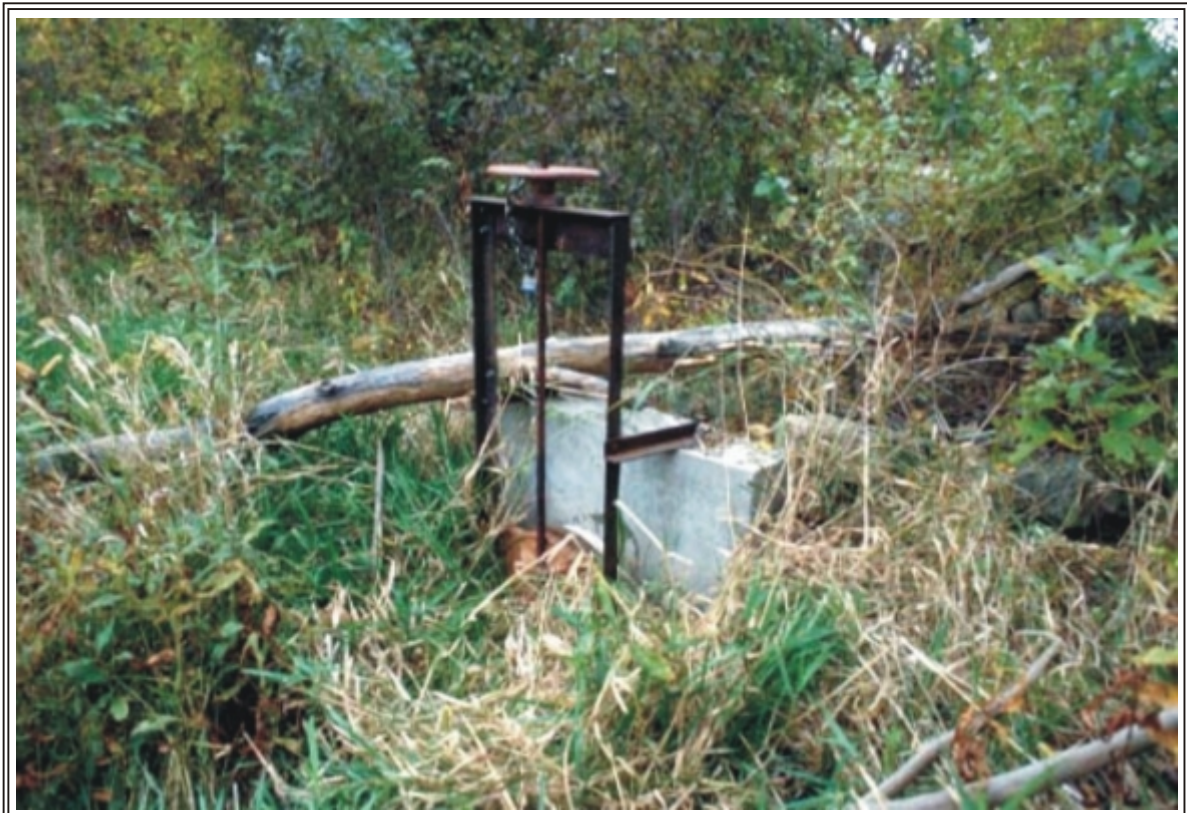
Figure 34. View Northeast at Water Control Structure #3.
