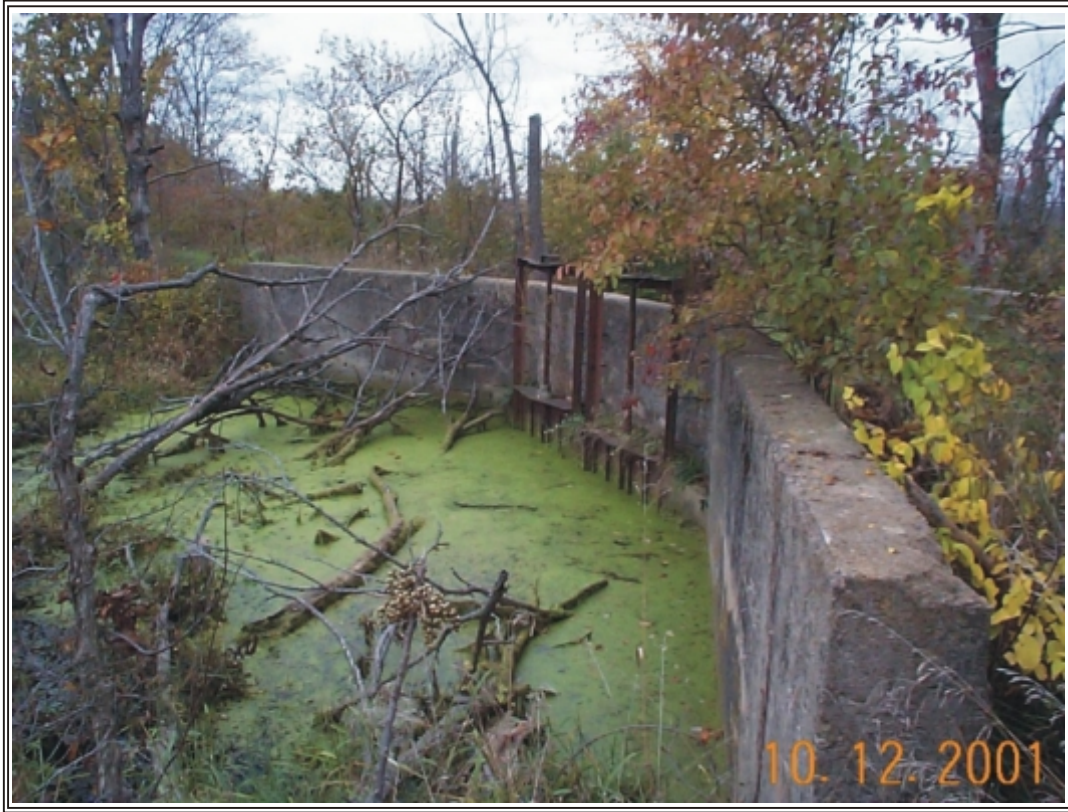
Figure 33. View Southeast at Water Control Structure #2.
